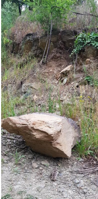
Unstable bank / falling rocks
